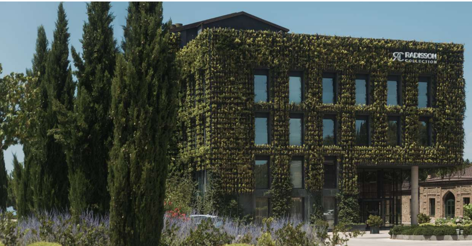
Views of the building
