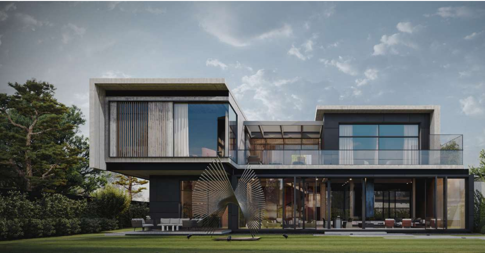
Views of the building
